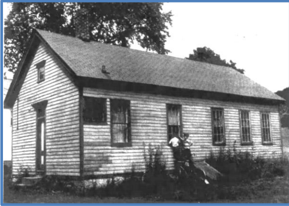
The Bradley Street School, c. 1970 from the Berkshire Eagle.
